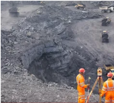
Mining and Civil Services
